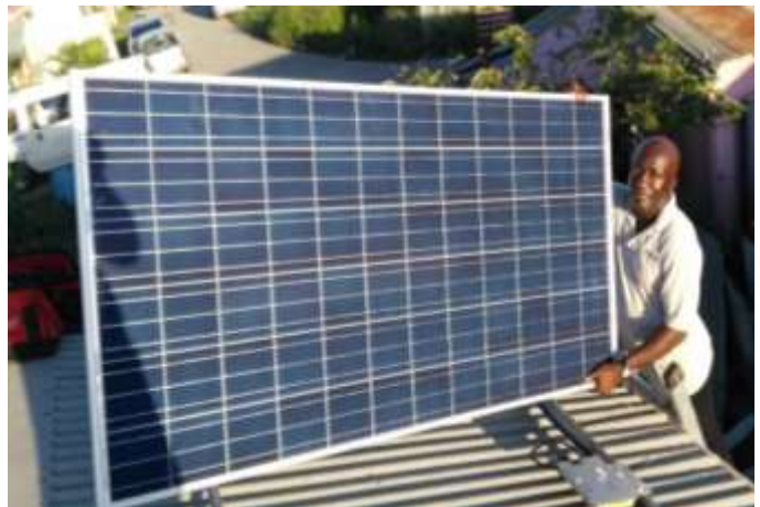
Antigua and Barbuda, 4 MW wind and solar project
